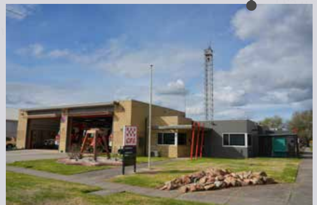
Current fire station
