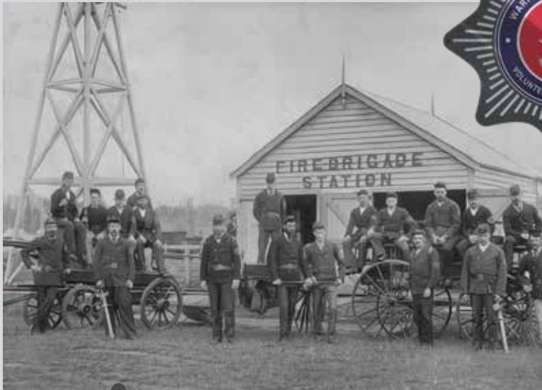
Original fire station, 1900s
