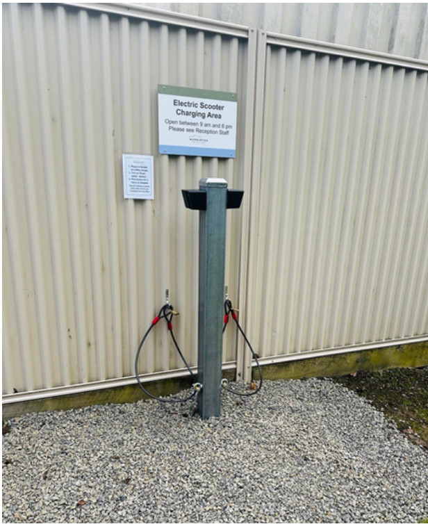
Personal light electric vehicle charging point at a caravan park. Note the bike locks to secure the LEV while being charged.
