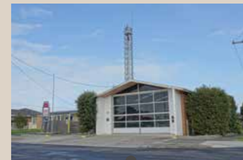
Current Yarram Fire Station
