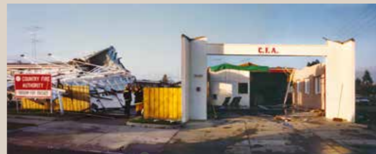
Station loses roof and hose tower in storm, late 1980s
