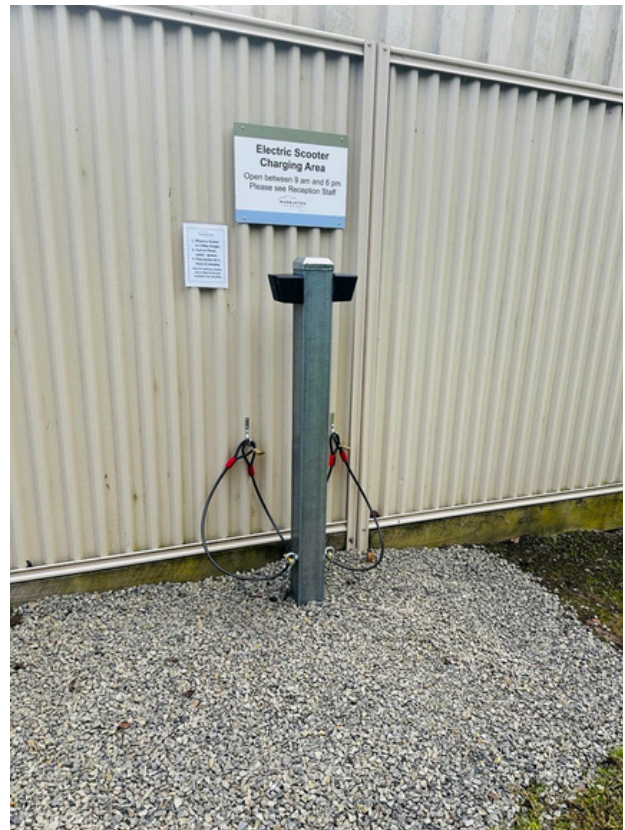
Personal light electric vehicle charging point at a caravan park.
