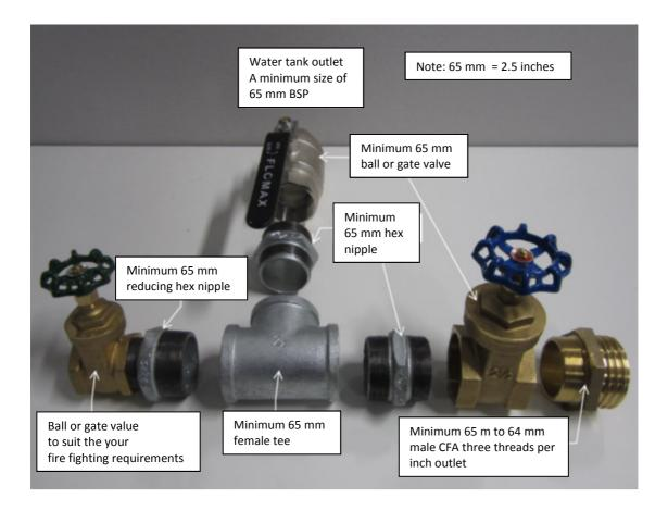
CFA FSG 006 - Tank connections explained - Bushfire Management Overlay
