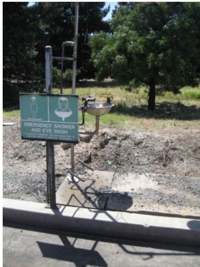
Photograph 4 Unlagged pipework and rough surface
