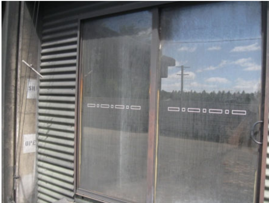
Photograph 5 Glass door on single storey fire attack building
