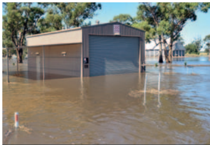
The Teddywaddy shed flooded again in January. Photo by Jenny Pollard
