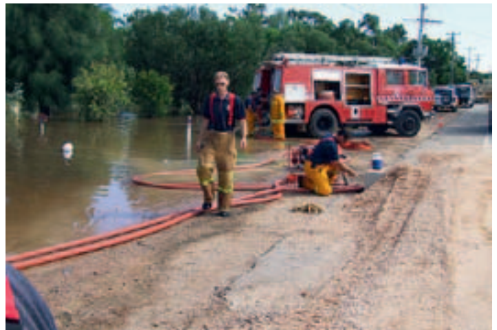
Working in the Hood Sector, several pumps, a tanker and a quickfill were able to shift 15,000 litres per minute from inundated houses. Photo by Steve Russell
