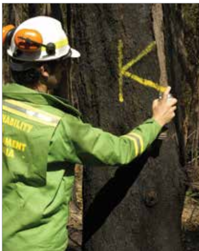
Figure 13 – qualified or experienced firefighter marking 'Clear and Present Danger' trees with a 'K'
