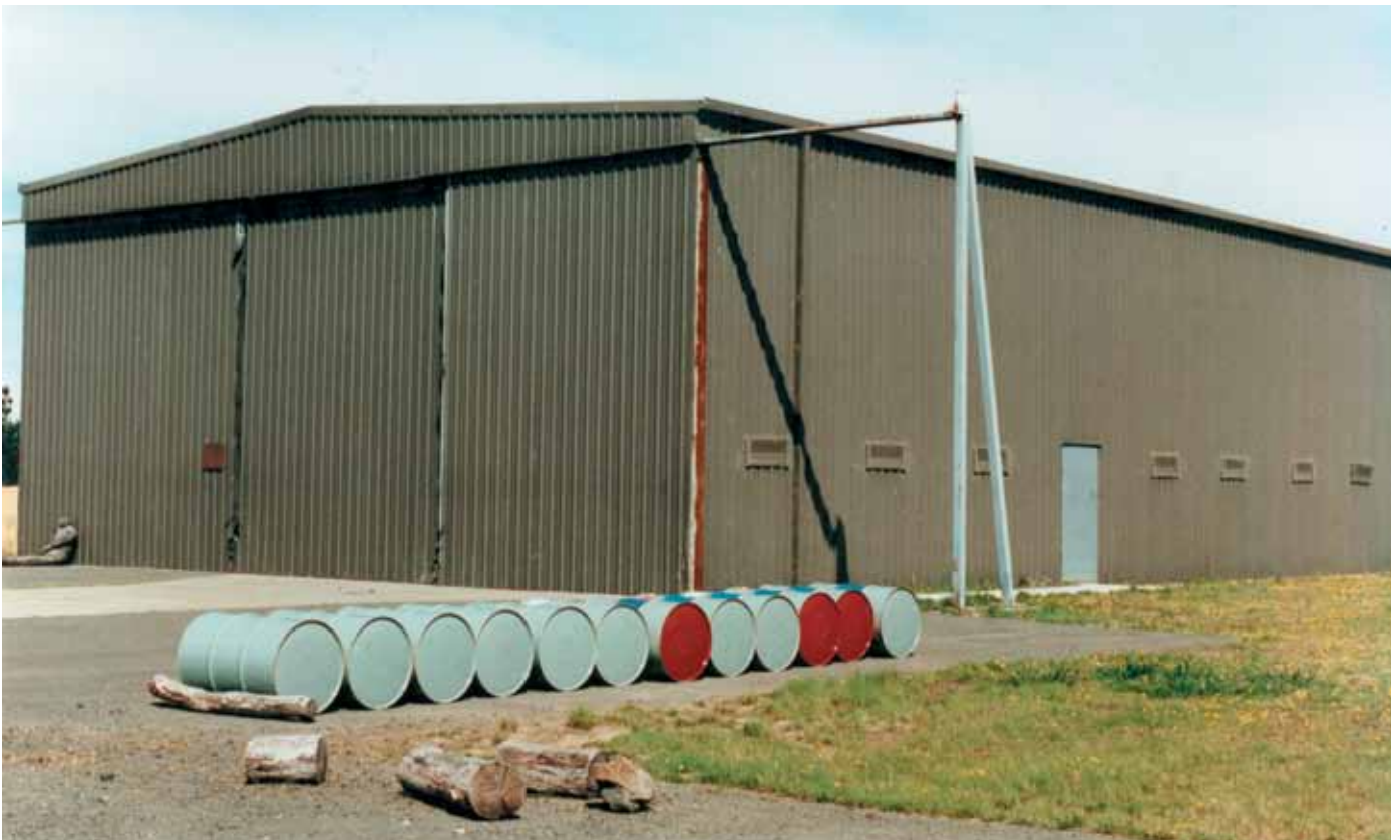
Avgas storage at Fiskville, non-compliance with Bureau of Air Safety, 1995/96. Photo courtesy of CFA
