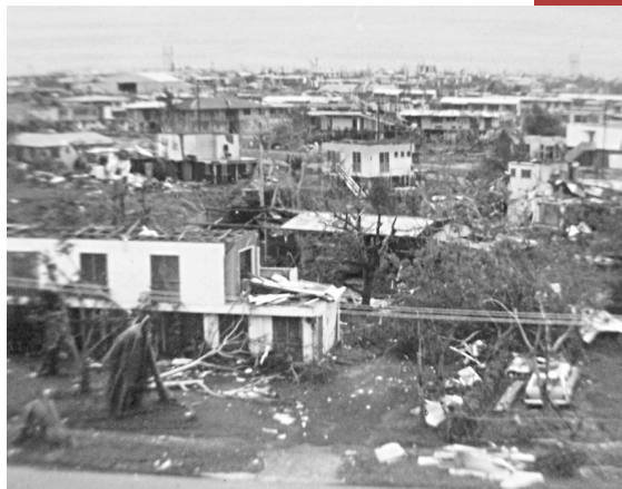
Damaged houses after the passage of Cyclone Tracy. Source: Wikimedia Commons
