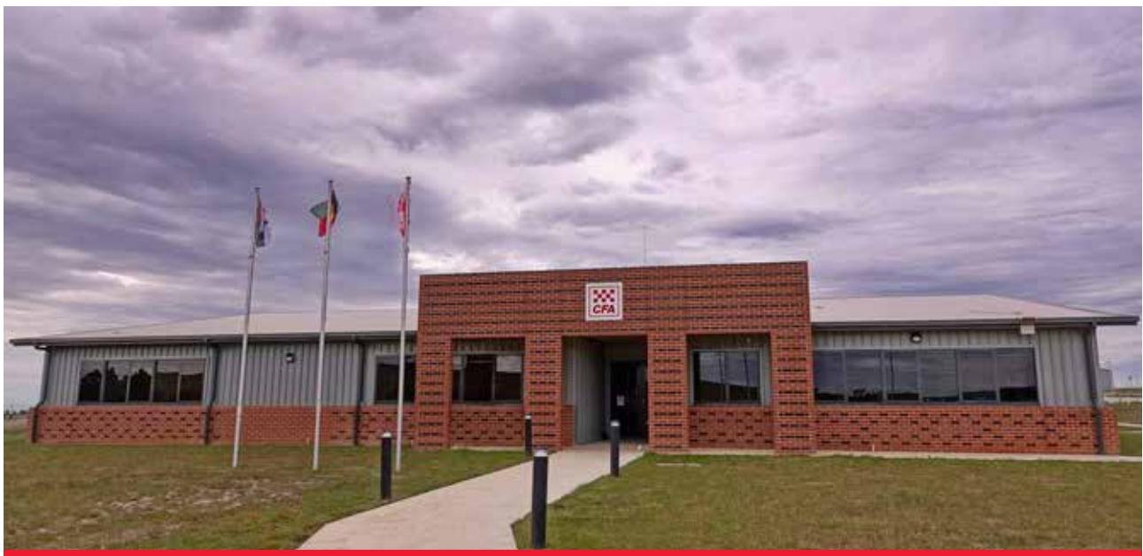
The new Central Highlands Regional Training Campus will open in 2021-22
